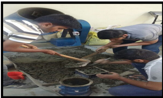
Figure 6. Casting of Specimens
