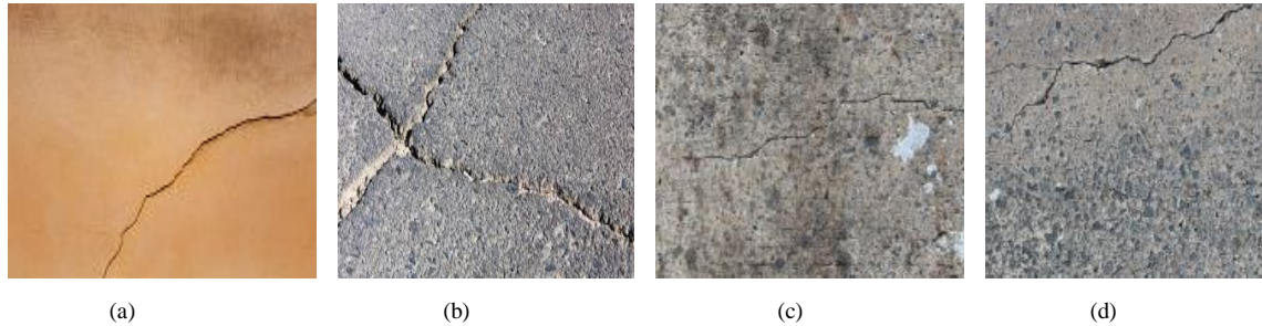
Fig.1. (a), (b) images that are with high contrast. Simple methods like edge detection and thresholding can be applicable to these images for crack detection.
