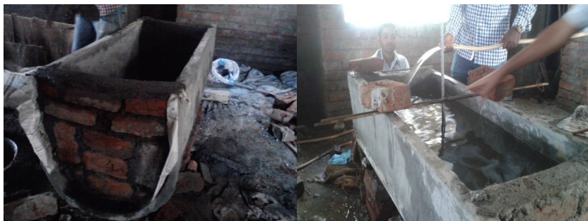
Photo 3.9 - Bund construction & Setup for leakage test.
