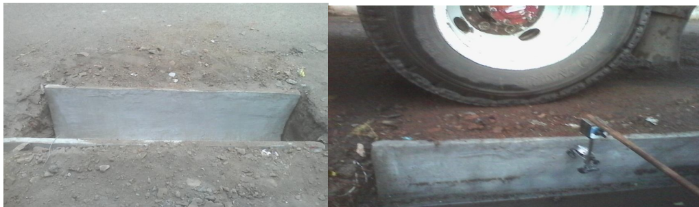
PHOTO 3.20 – Placing of gutter & Deflection test.
