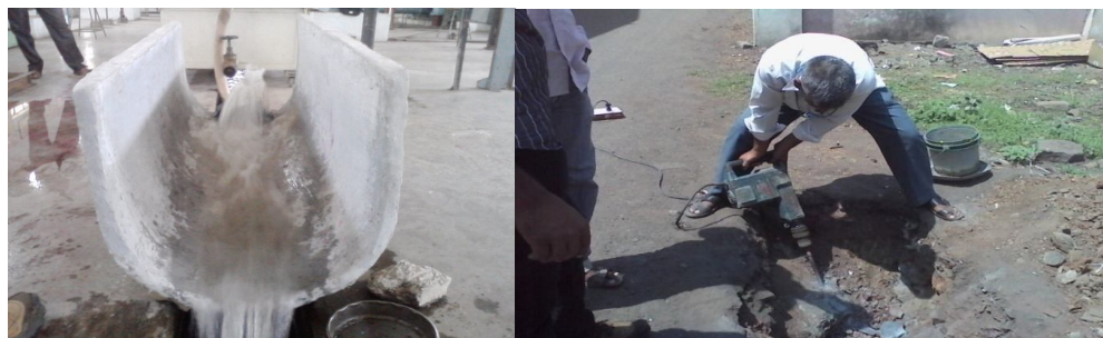
PHOTO 3.18 – Scouring test & excavation
