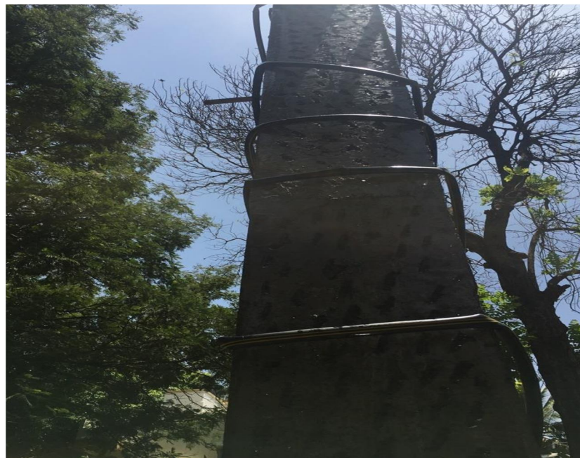
Figure no 6:- drip curing applied to a column on site
