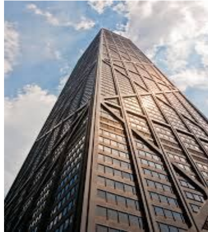
Fig.1 Braced tube structure (John Hancock Center)
