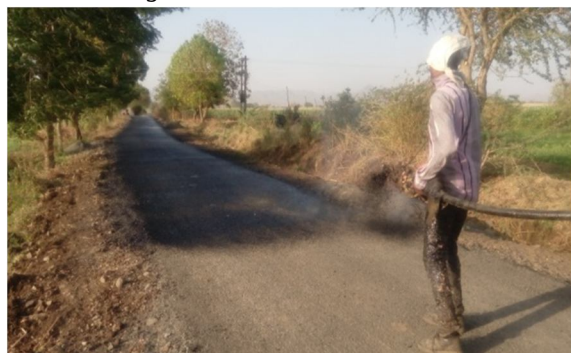
Fig-4 Bituminous mix lying on site
