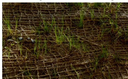
Fig. 13: Vegetation Canopy on the Jute Geotextile
