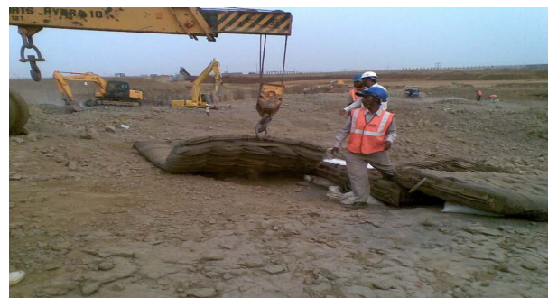
Laying of blasting pads by hydra
