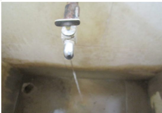
Fig 2: Water Leakage after tap is closed.
