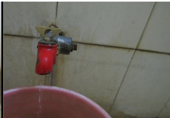
Fig 3: Water Leakage after tap is closed.
